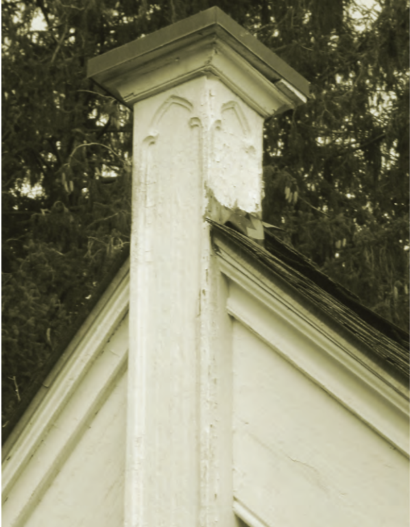
King post built to match the existing architectural detail on an extension to the original building.
