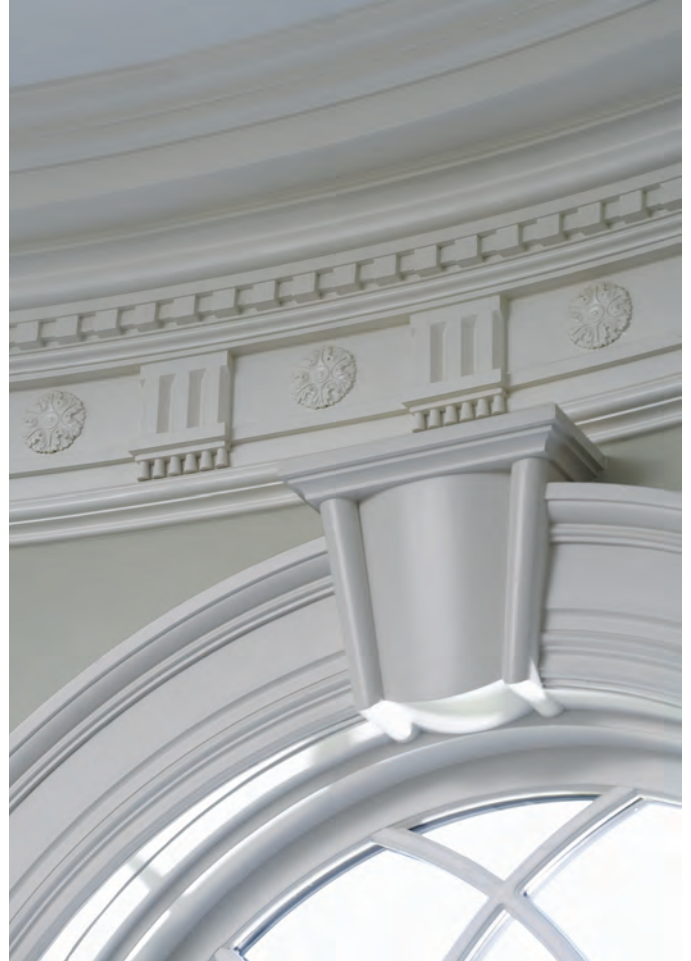
Key block on custom curved cased window with compound crown above.
