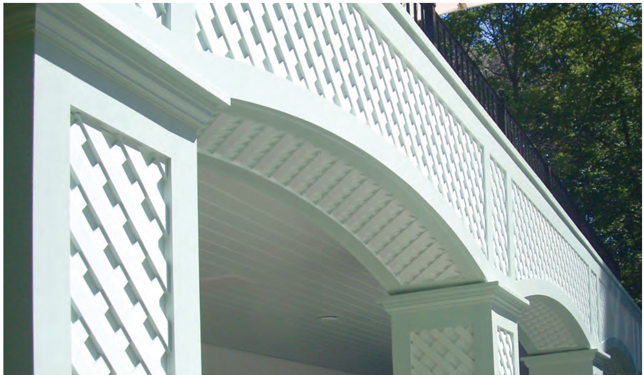
Custom Cellular PVC trellis work was a perfect complement to a pool area where moisture is commonplace.
