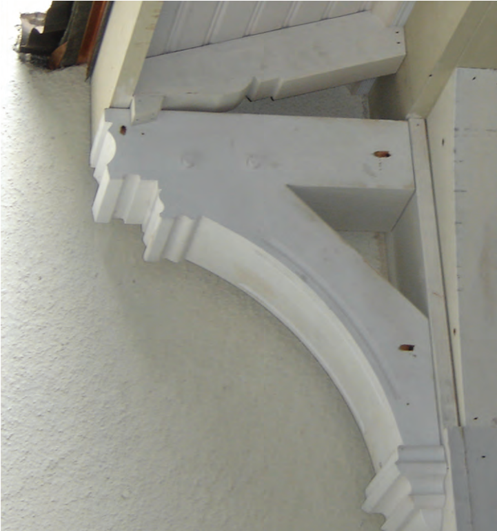
Ornate bracket built to replace the original architectural detail.
