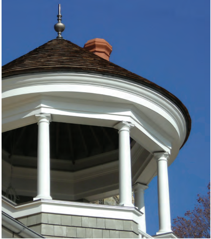
Custom curved exterior trim produced in AZEK®.
