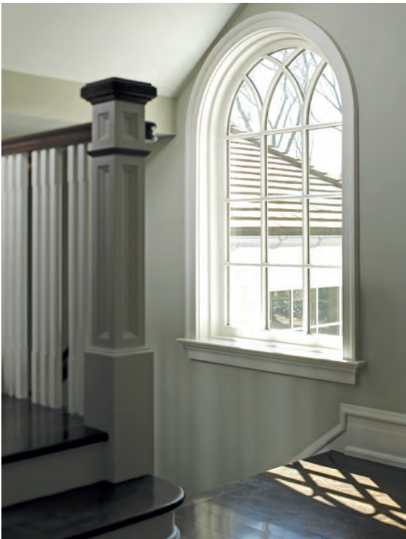
Curved casing wraps this arch top window.
