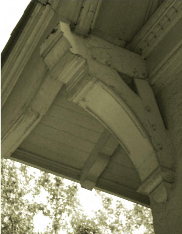
Ornate bracket built to replace the original architectural detail.
