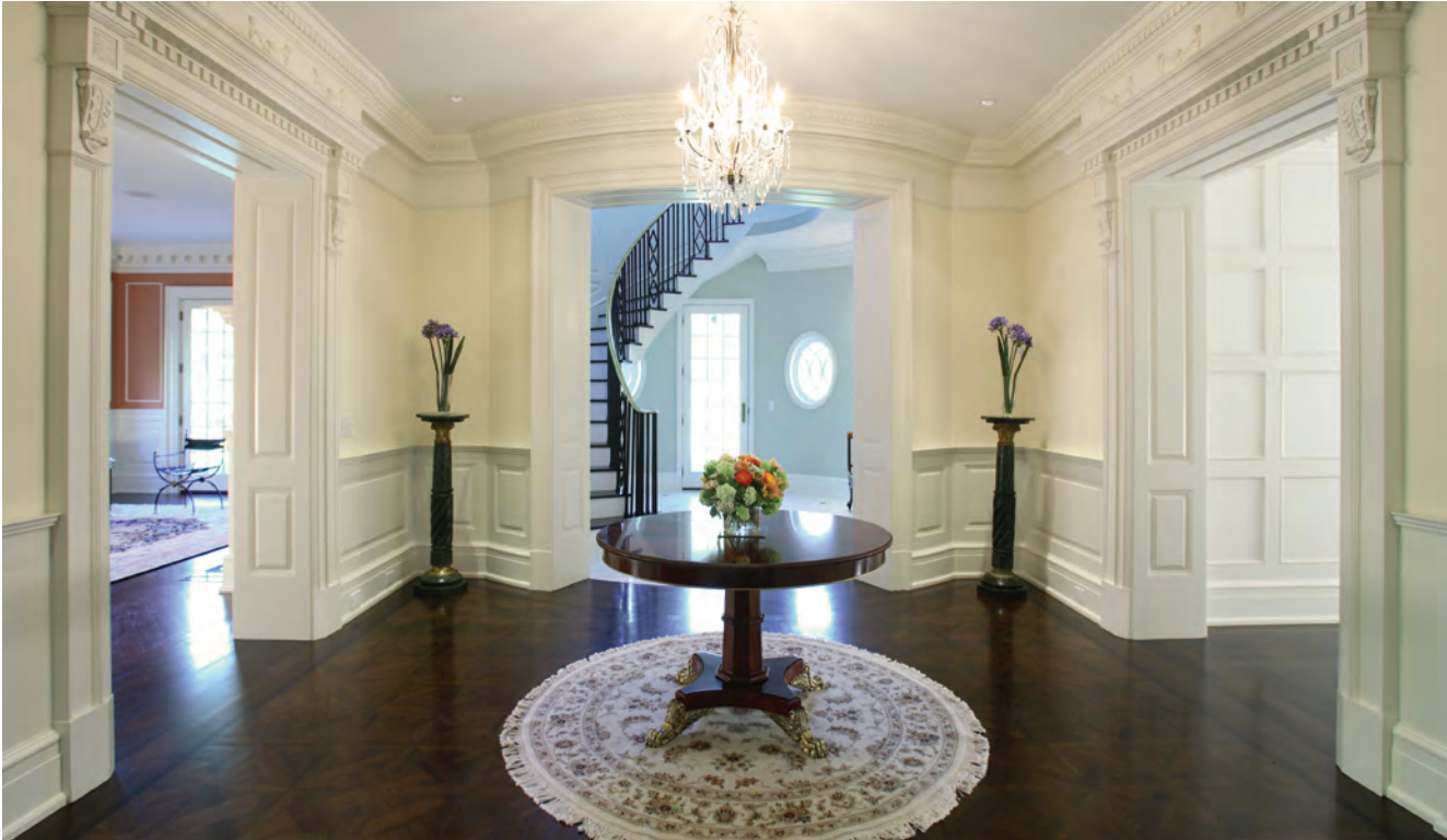
Elegant foyer with curved panels, casings and crowns.
