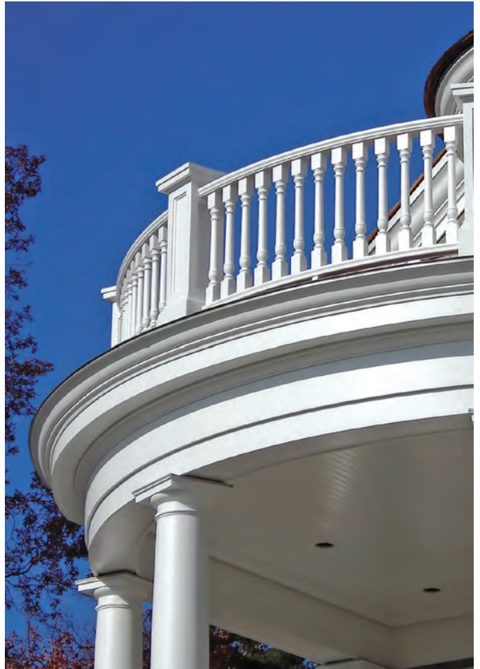
Cellular PVC is an ideal material for radius work, as seen on this balcony.
