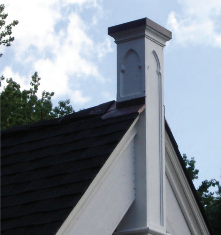
King post built to match the existing architectural detail on an extension to the original building.
