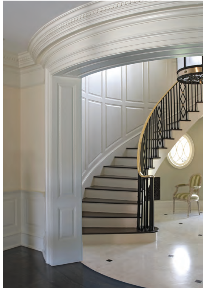
Curved cornice and paneled jamb lead to curved stairwell.
