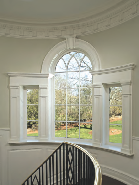
Curved cornice, window and casing on curved stairwell.
